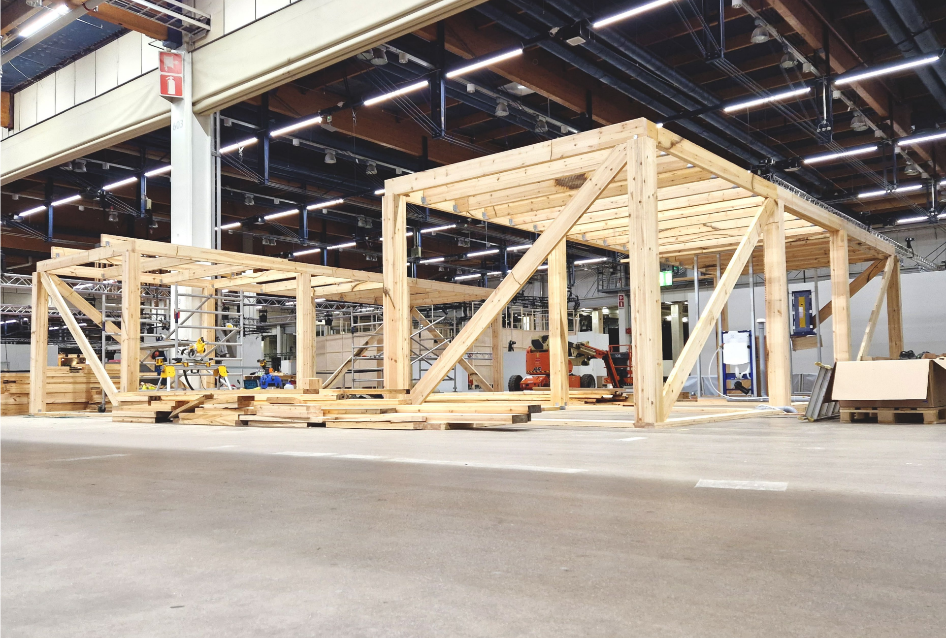
Collecting and refining the chosen materials: Reused glulam timber structures as beams and columns of a frame of an exhibition building.
